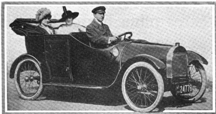
Two views of the new Twombly taxicab to sell for $600. The passengers have an unobstructed view because the driver sits in the center
